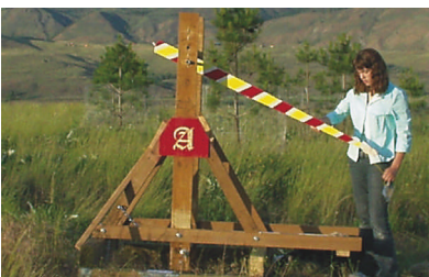
Figure 1 Allie inspects her beam for damage.
